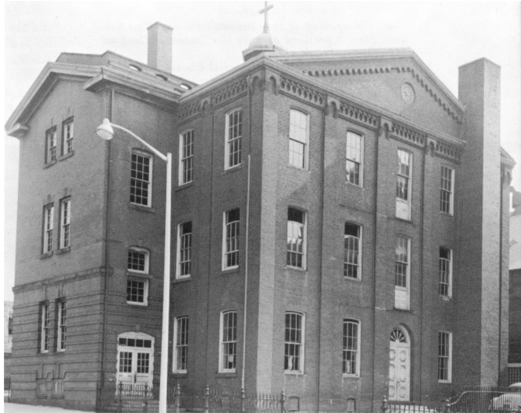
ST. PAUL'S SCHOOL-PRESENT EXTERIOR
