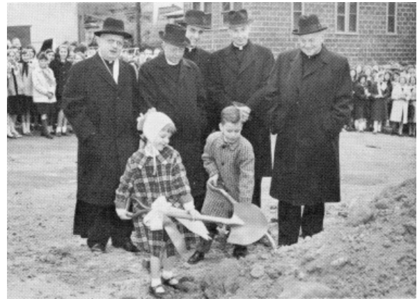
GROUND BREAKING FOR NEW SCHOOL
